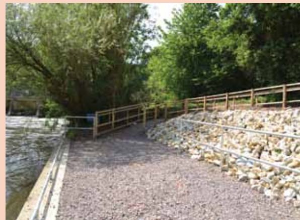
Neither fish nor fowl: Interim stage before the surface stones were removed, ramped access and level fishing area established
