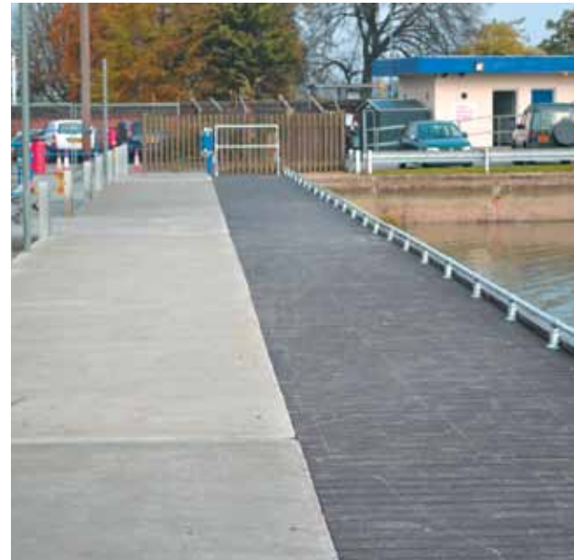
This large group platform in London is made from recycled plastic with a non-slip surface
