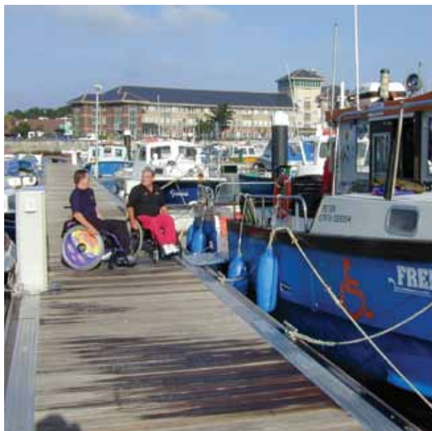
Wide, level and non-slip approaches help to facilitate access onto boats
