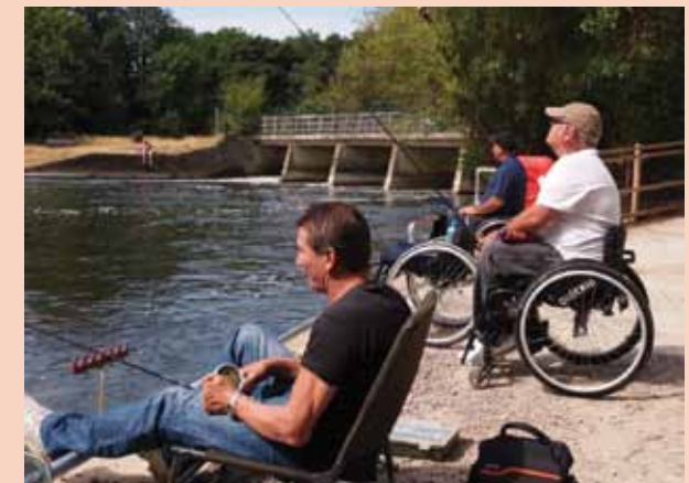
A good catch: The final accessible platform has a smooth finish made from a fine concrete and sand mix
